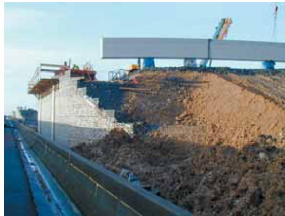
Photo 5 Culée Terratrel Terratrel abutment
