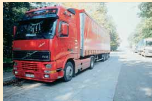
A6 - Aire des Châtaigniers (rest area) : commercial vehicle parking lot of thin bonded concrete overlay
