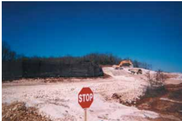
Photo 9 Film de protection de la station botanique d'hélianthes (A20 T3.3) Protective film for the botanical station for rock-roses (A20 T3.3)
