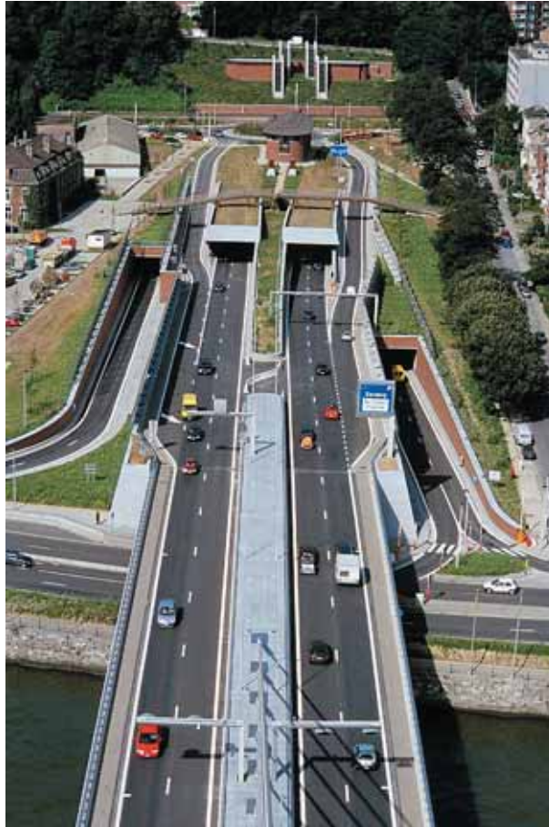
Photo 2 Tête "Tilleuls" des tunnels de Cointe "Tilleuls" head of the Cointe tunnels
