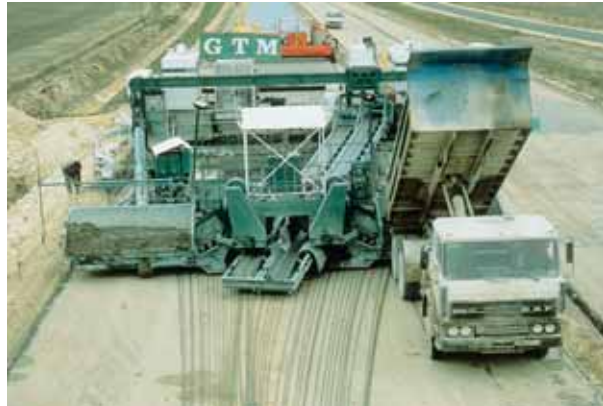
Photo 1 BAC : chantier de l'autoroute A71 Continuous reinforced concrete : A71 motorway project
