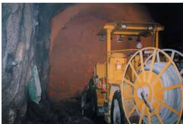
Photo 7 Foration de la volée Drilling the blasting holes
