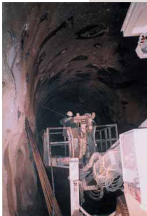
Photo 9 Boulonnage Rock bolting
