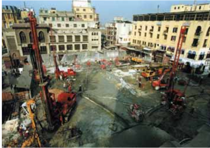
Photo 7 L'hydrofraise à Port Said en action The hydro-cutter in action at Port Said
