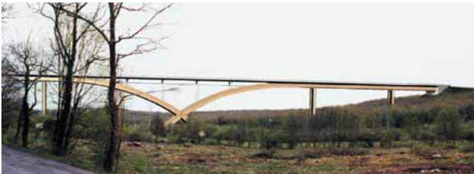
Photo 7 Tirants aériens Aerial tension members
