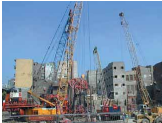
Photo 7 L'hydrofraise à Port Said en action The hydro-cutter in action at Port Said
