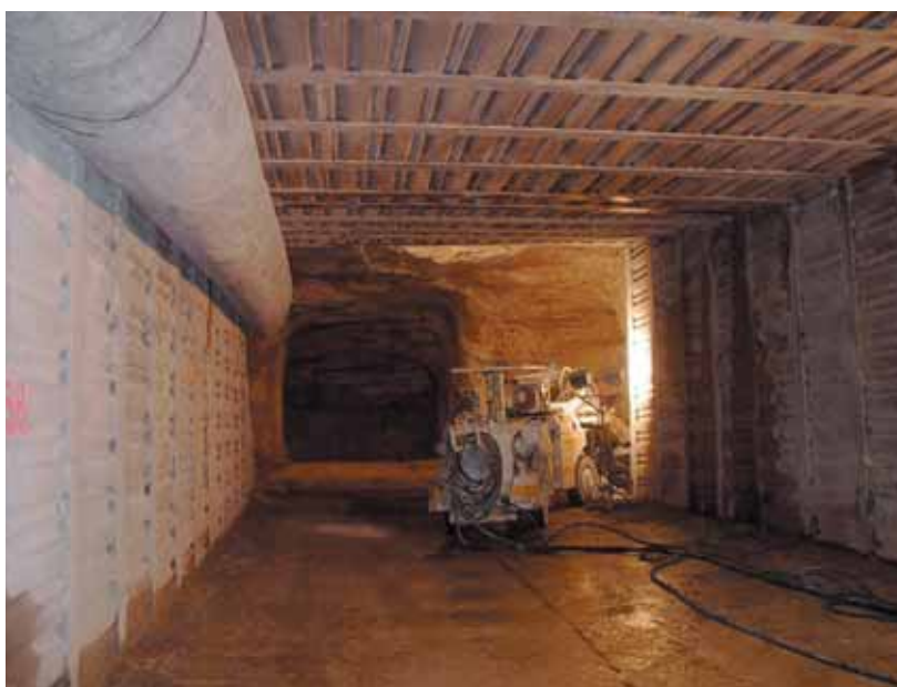
Photo 3 Soutènement Supporting structures
