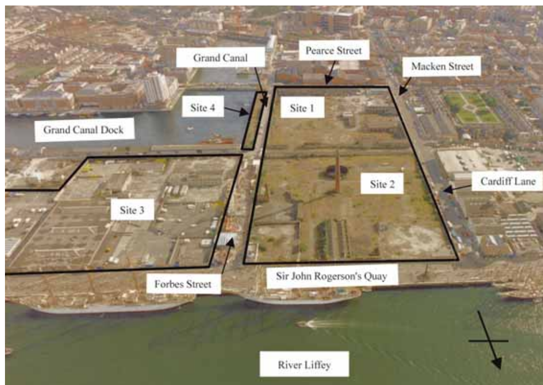
Plate 1 Aerial view of Sites 1 to 4 prior remediation works
