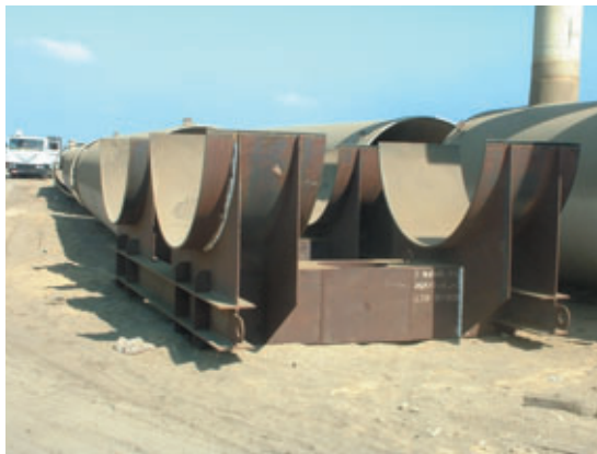
Photo 9 Berceaux de support des tuyaux GRP Support cradles for GRP pipes
