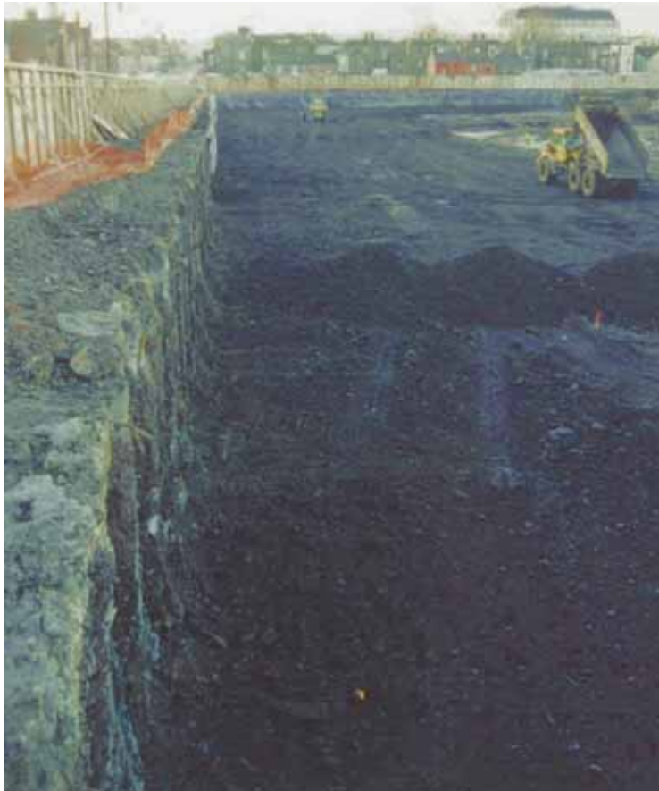
Plate 2 Photograph of exposed hybrid wall
