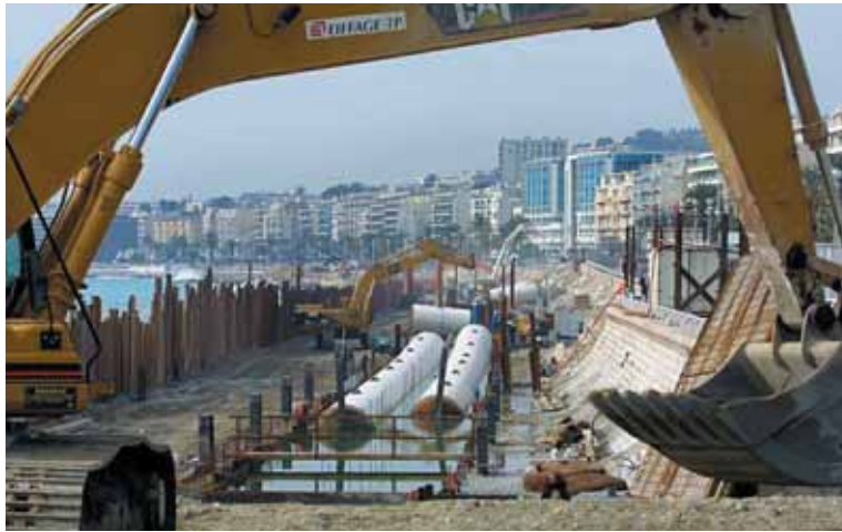
Photo 5 Lancement des tuyaux Launching the pipes
