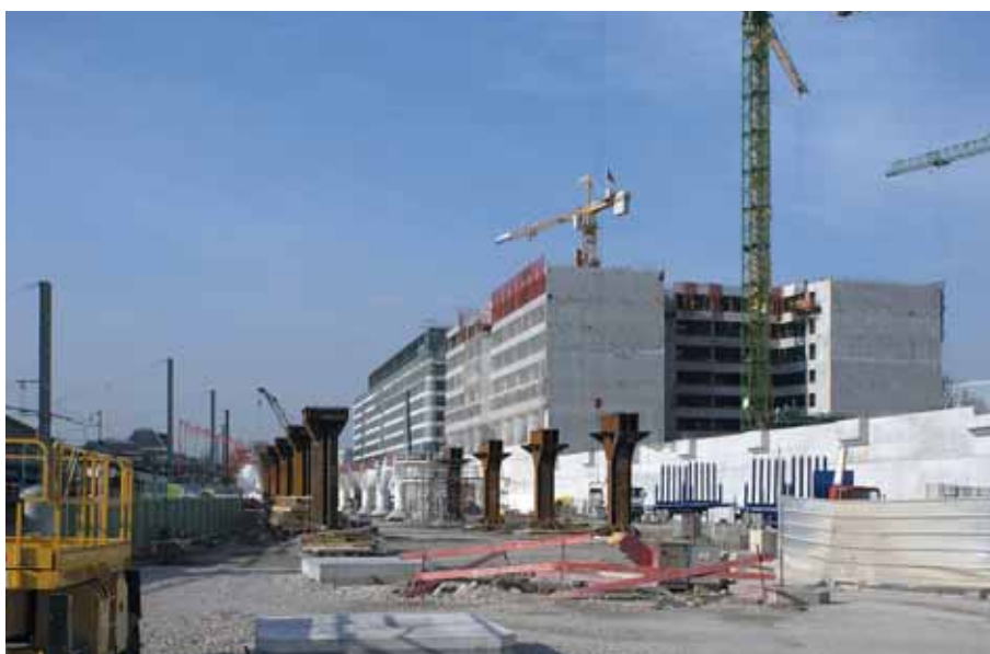
Photo 7 Coactivités des chantiers Co-activity on construction sites
