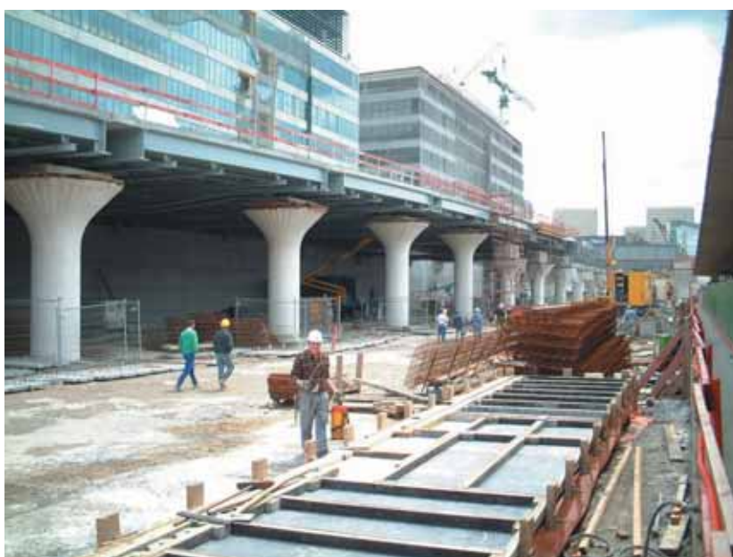
Photo 1 Exemple de structure mince Example of thin structure
