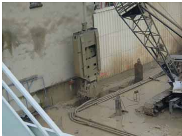
Photo 3 Excavation le long des mitoyens Excavation along the adjoining buildings
