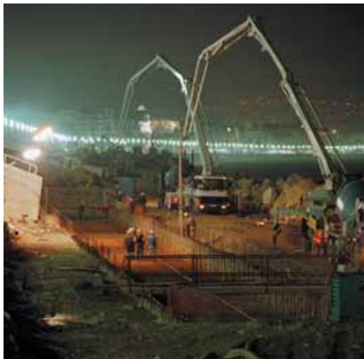
Photo 6 Bétonnage de nuit Concrete by night
