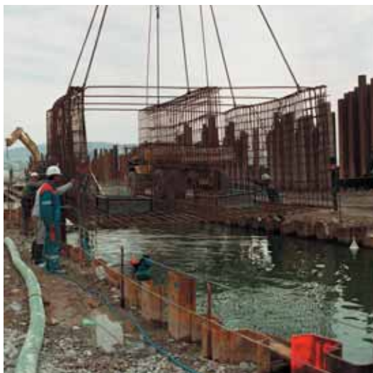
Photo 4 Cage d'armatures Concrete reinforcing cages
