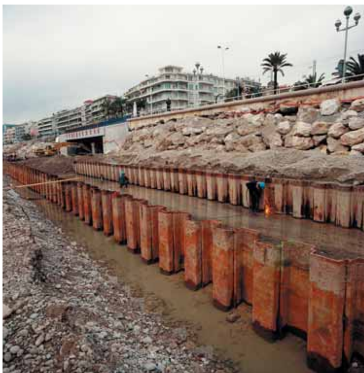
Photo 8 Recépage palplanches Cutting off sheet piling
