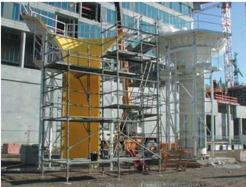
Photo 3 Coffrage des poteaux architecturaux Shuttering of architect-designed columns
