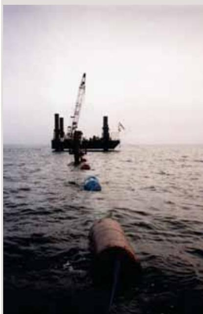
metres long, to permit crossing of a protection dyke. The route followed by the outlet is 40 % in sound limestone rock.
