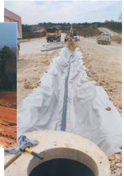
Photo 6 Pose de drains Drain laying
