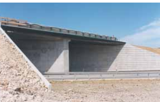
Photo 8 Pont-route à Azerat Road bridge at Azerat
