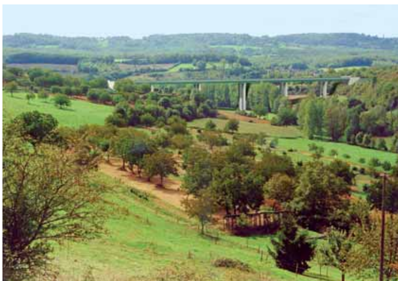
Photo 1 Vue du nord (montage) North view (assembly)
