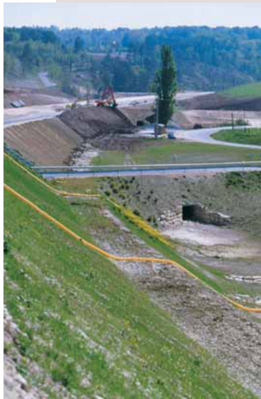
Photo 11 Talus engazonnés Earth banks planted with grass
