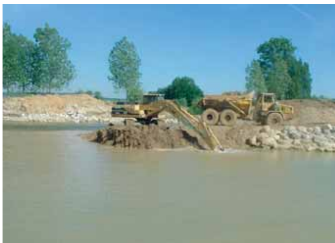
Allan : reprise batardeau aval Allan : repair of cofferdam downstream
