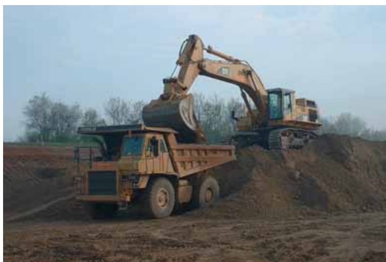
Photo 2 Atelier type terrassement Typical earthworks equipment
