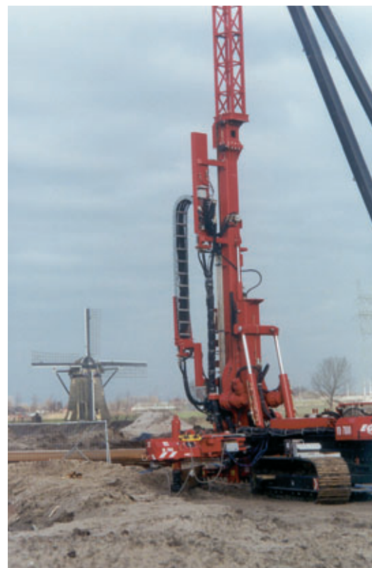
Photo 7 La foreuse de jet grouting The jet grouting drill
