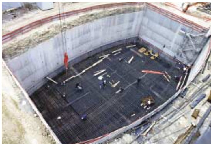
Photo 2 Le radier The foundation raft
