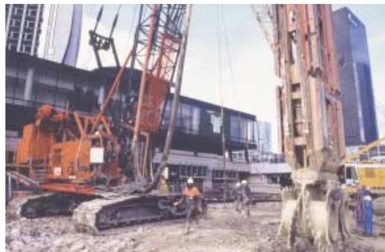
Photo 3 Hydrofraise Hydrofraise drilling machine
