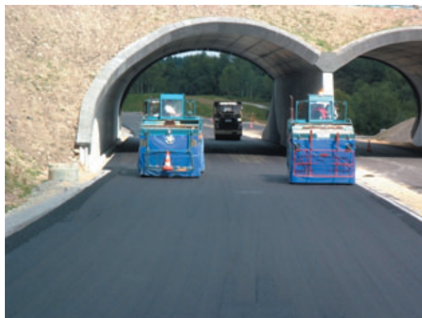
Compactage de la couche de roulement Compacting the wearing course
