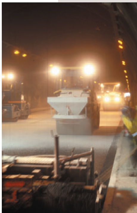
Photo 4 Compactage de Lumichape Lumichape compacting
