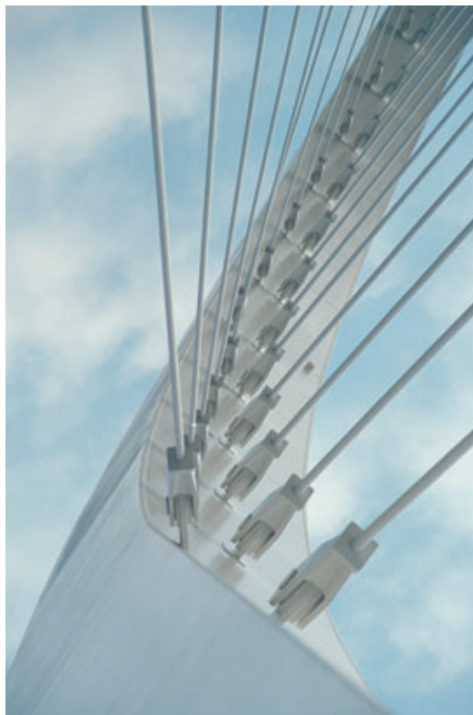
Photo 5 Attache des suspentes sur l'arc Attachment of suspenders to the arch
