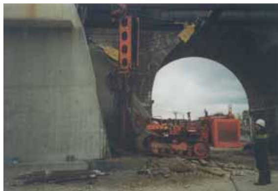
Injection on piers - Pier peripheral breakwaters, later permitting access to the pier heads for the reworking and demolition stages
