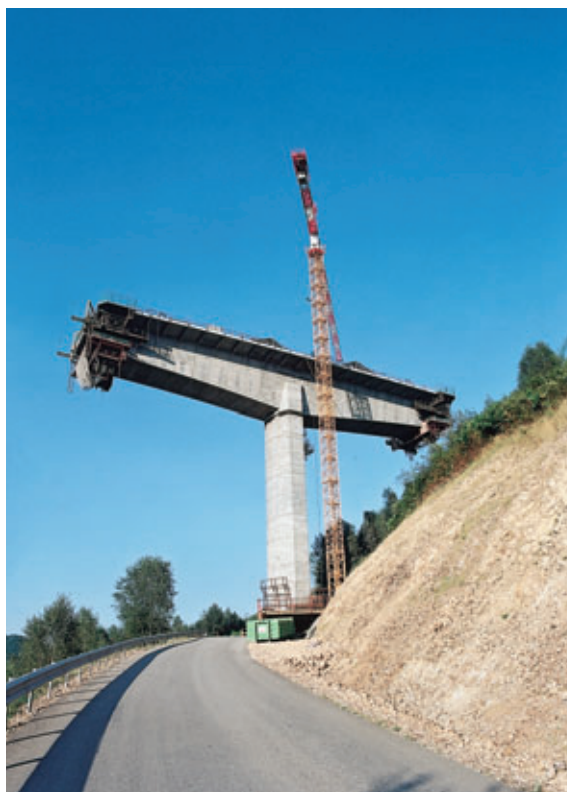
Photo 3 Fléau n°5. Equipages mobiles. Encorbellements Beam No. 5. Mobile rigs. Cantilevering
