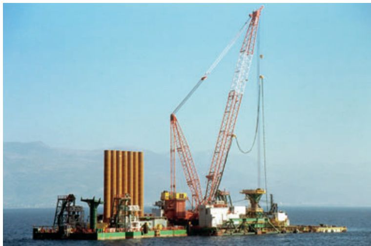
Photo 2 Lisa et le catamaran en cours de battage Lisa and the catamaran during driving
