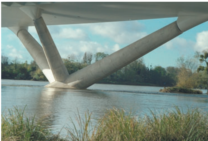
Photo 6 Les piles tripodes Tripod piers
