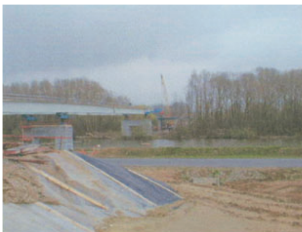
Photo 9 Lancement de la charpente Launching the structural work
