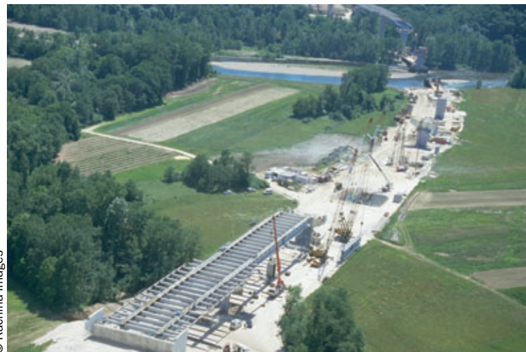
Photo 2 Elévation de l'ouvrage Elevation view of the structure
