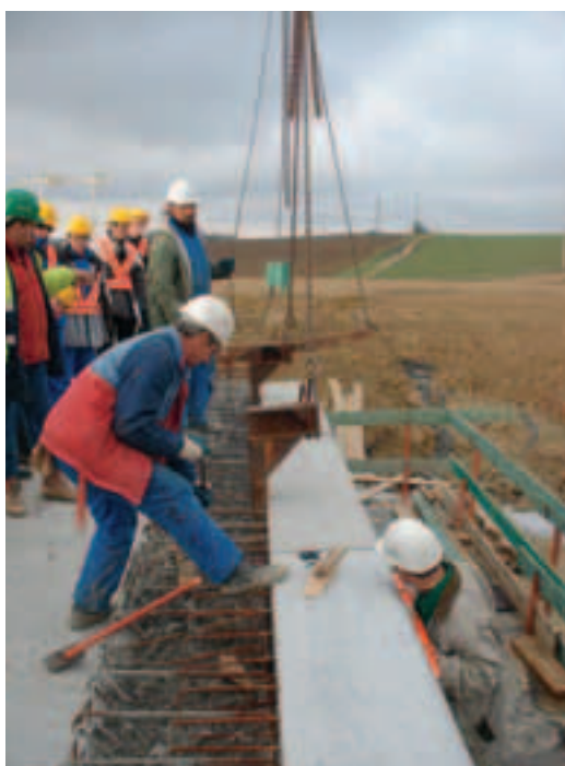
Photo 10 Pose de corniches Placing of cornices
