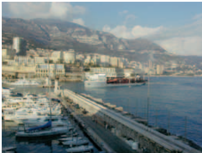
Photo 1 Drague "Nile River" "Nile River" dredge
