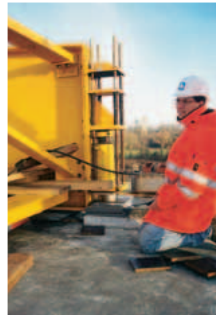
Photo 5 Relevage de l'avant-bec lors de l'accostage Lifting of cutwater during positioning
