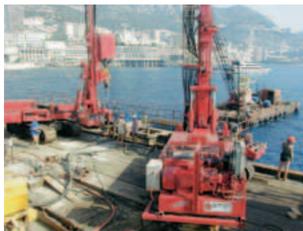
Photo 3 Injections solides - Perforatrices Solid injection - Drilling rigs
