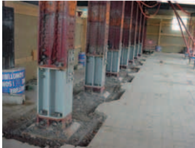
Photo 5 Ouvrage existant relevé Existing bridge raised
