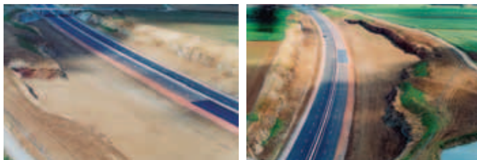
10 – 11 Traitement d'un emprunt. A28 – Scao – Socaso – Cofiroute A borrow zone. A28 motorway – Scao – Socaso – Cofiroute
