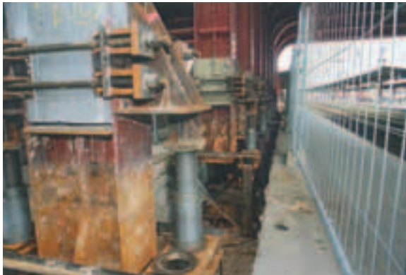
Photo 4 Relevage de l'ouvrage existant Raising of existing bridge
