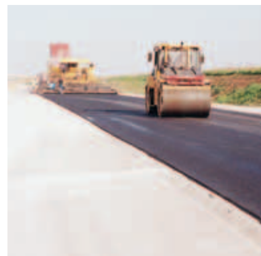
Photo 8 Compactage du sable enrobé Compacting of treated sand
