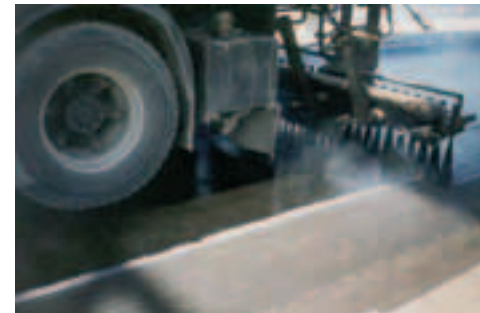
Photo 6 Application de la membrane Evatech LD Application of Evatech LD membrane
