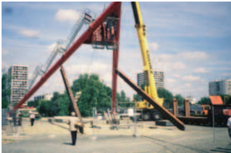
Lifting one of the two steel towers
