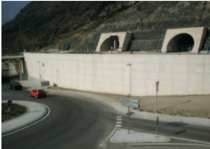
Photo 8 Tête sud du tunnel South head of tunnel
