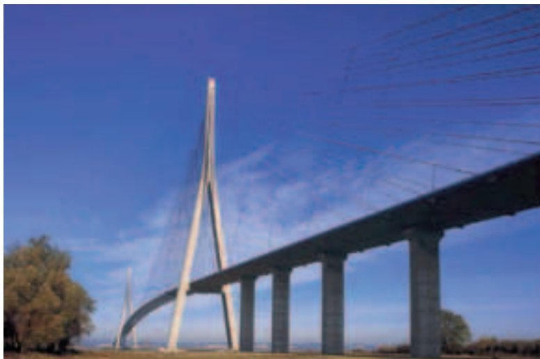
Photo 6 Scanprint™ "observe" les haubans du pont de Normandie Scanprint™ "observes" the stay cables of the Normandy Bridge
