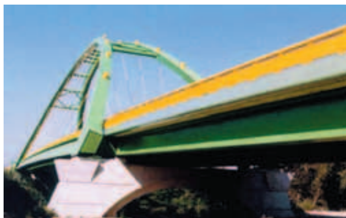
Photo 2 Pont de Saint-Gilles Saint-Gilles Bridge
