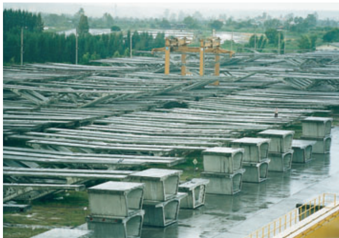
Figure 16 D6 storage Stockage D6
