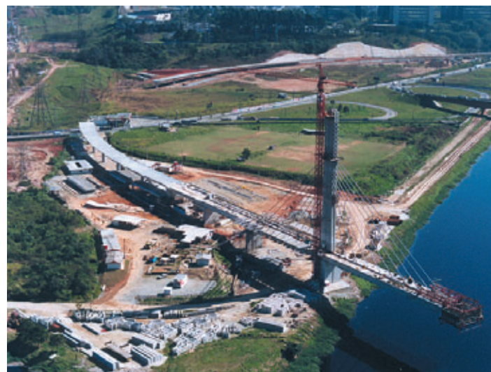
Photo 2 L'ouvrage en construction Structure during construction
