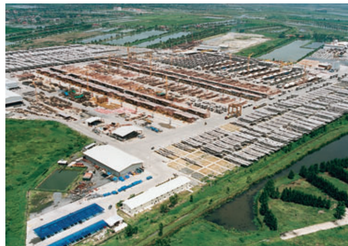
Figure 6 Precast yard Bang Po
