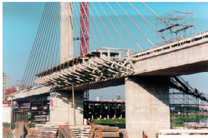
Photo 6 Les fermes support des quais Platform support frames
