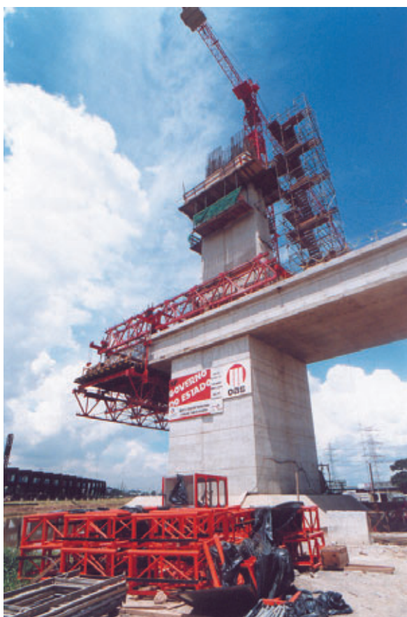
Photo 3 Le pylône The tower
