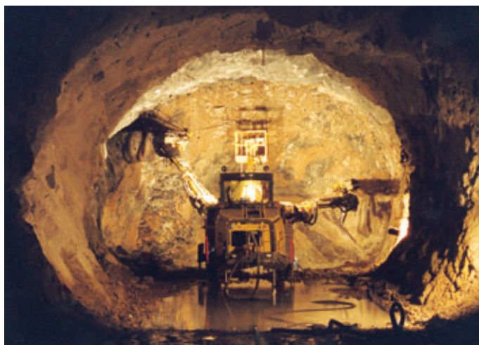
Photo 2 Excavation Jumbo Atlas Copco L2C Excavation : Jumbo Atlas Copco L2C
