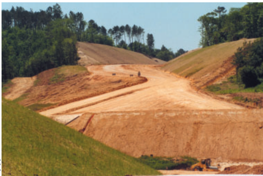
Photo 13 Terrassements sur Montpon/Mussidan Earthworks on Montpon/Mussidan section
