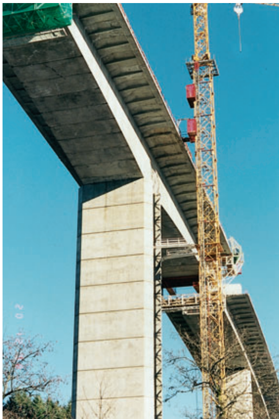
Photo 8 Equipage mobile en phase de déplacement Travelling formwork being moved
