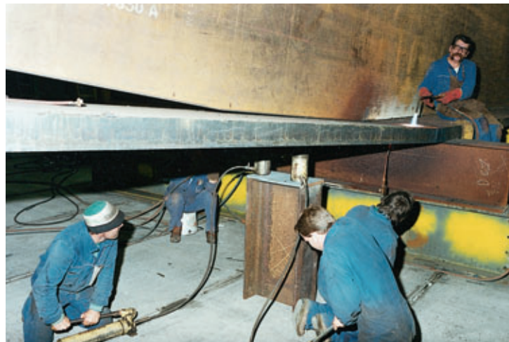
Photo 1 Forgeage de la semelle inférieure Preparing the lower footing
