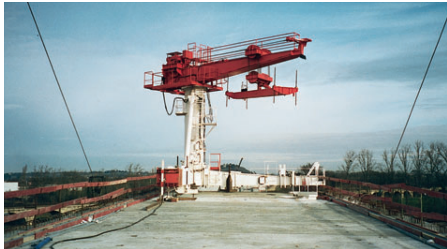
Photo 5 Potence de pose Segment placement crane
