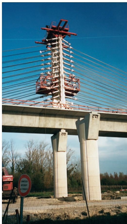
Photo 4 Mât de haubanage Stay post
