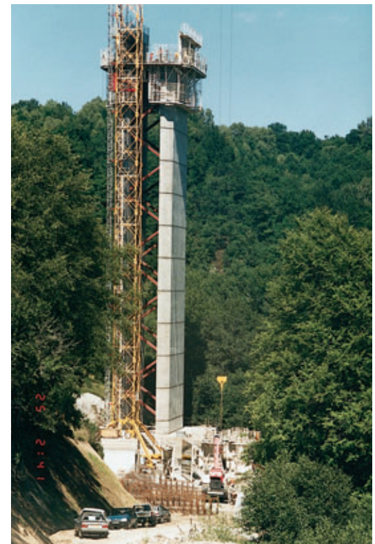
Photo 4 Pile P2 en cours de construction Pier P2 during construction
