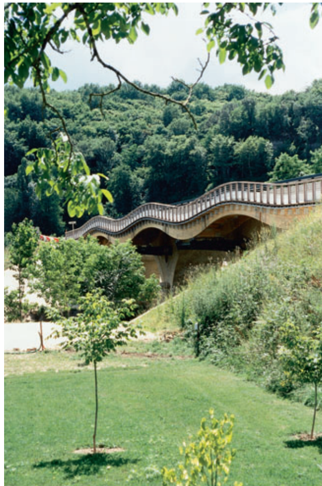
Vue aval d'ensemble de la passerelle Overall downstream view of footbridge
