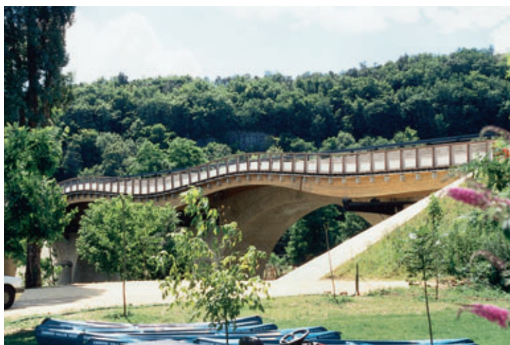
Vue aval de la passerelle Downstream view of the footbridge
