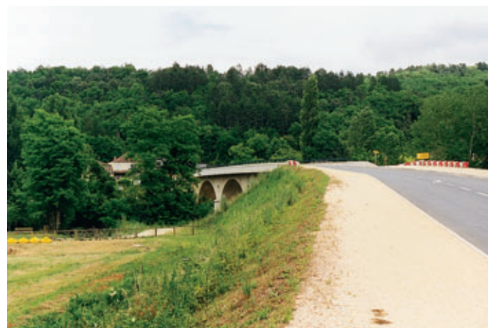
Vue amont Upstream view
