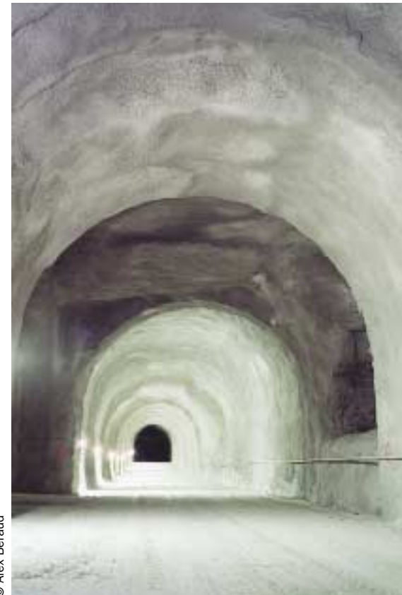
Galerie recalibrée et soutenue de raccordement à l'exploitation Re-sized and supported operational connection gallery
