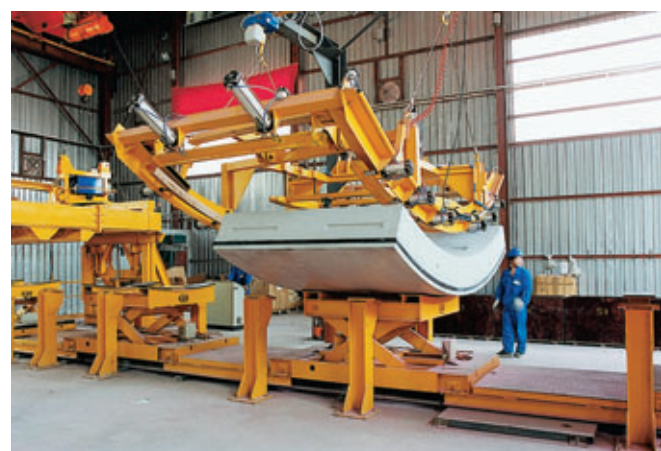
Photo 12 Usine de préfabrication - Encollage des joints Pre-casting plant - Gluing of joints
