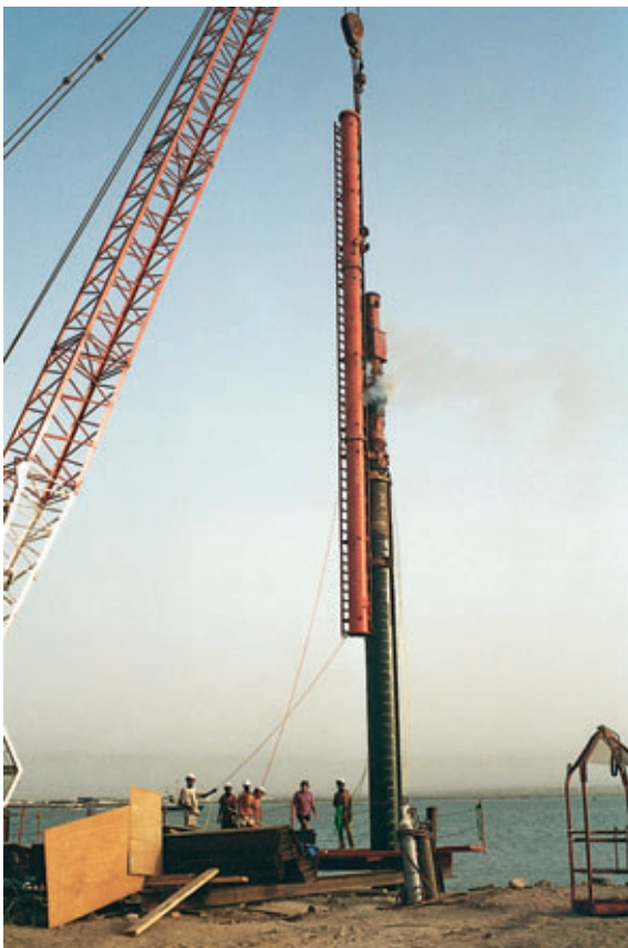
Photo 7 Battage Pile driving
