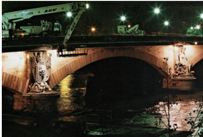
Photo 7 Travaux pont des Invalides Works on Invalides Bridge
