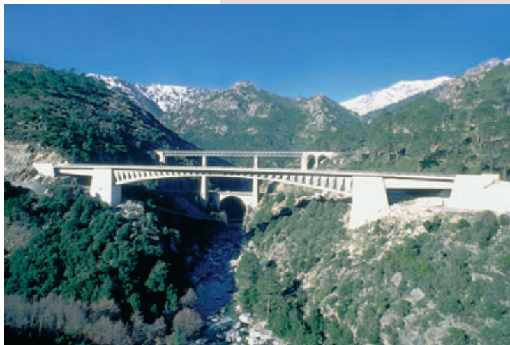
View of the three structures
