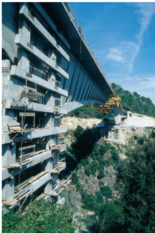
Photo 3 Poutre habillage P1 Beam - Trim P1
