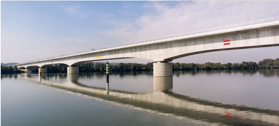
L'ouvrage terminé The completed structure
