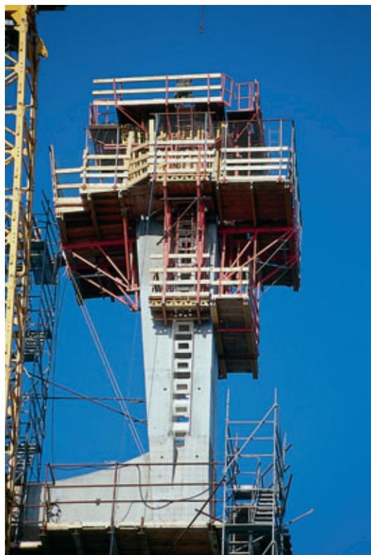
Photo 4 Coffrage pylône Tower formwork
