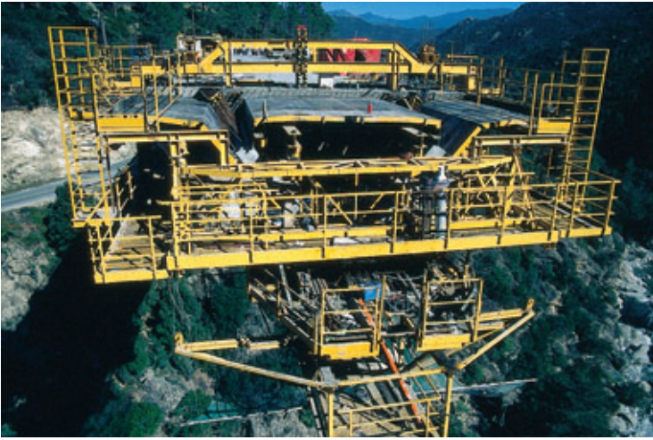
Photo 12 Equipe mobile Travelling formwork
