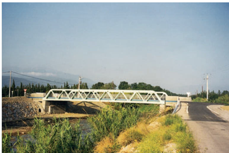
Ouvrage terminé Completed structure
