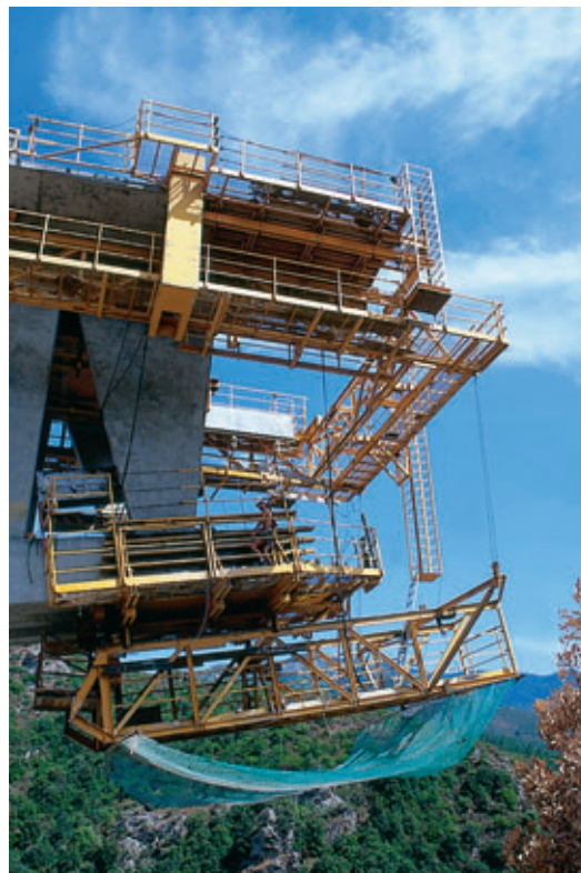
Photo 11 Equipage mobile Travelling formwork
