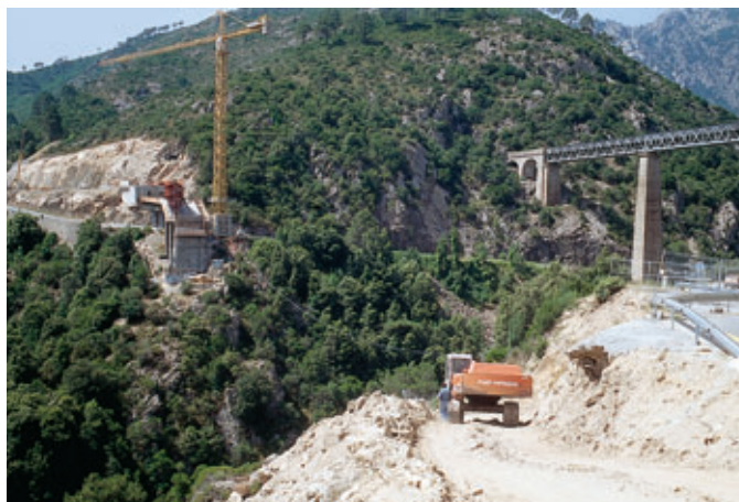
Photo 8 Terrassements pile P2 Earthworks pier P2
