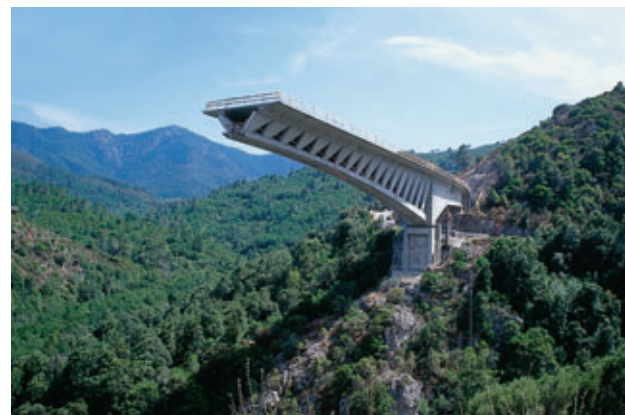
Photo 4 Fléau sud terminé South arm completed
