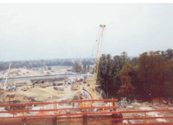
*Configuration of the Rueil-Malmaison worksite south of highway RN 13. Drilling for berlin-type walls, diaphragm walls, earthmoving and stock reclaiming. A noise barrier can be seen along the edge of the Petite Malmaison park*
