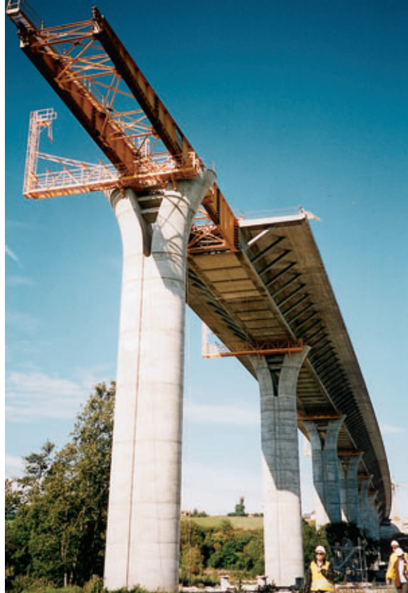
Photo 7 Le tablier en cours de poussage The deck during pushing
