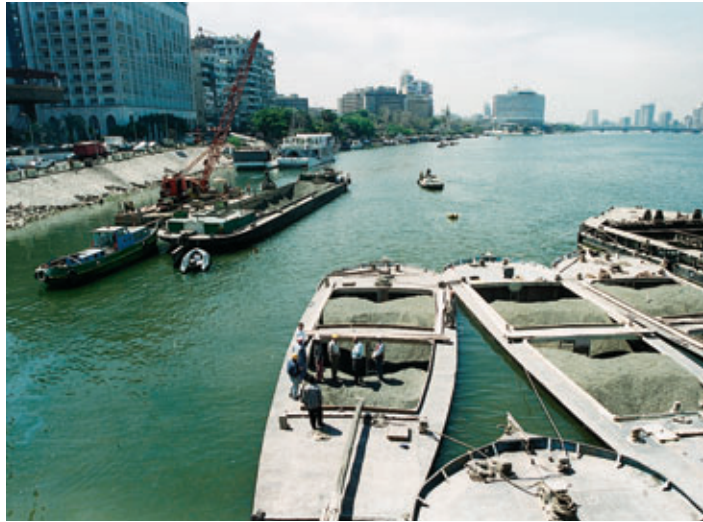
Photo 5 Travaux fluviaux de rechargement River build-up works
