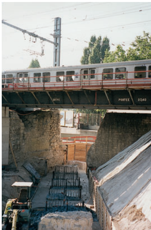
Photo 2 Tabliers auxiliaires en place Auxiliary decks in place
