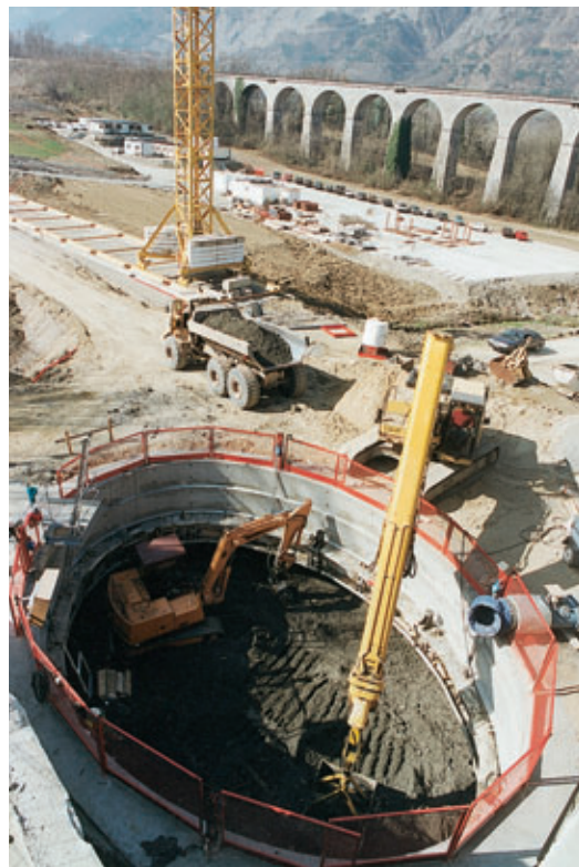
Photo 2 Excavation d'un puits marocain Excavation of a Moroccan shaft
