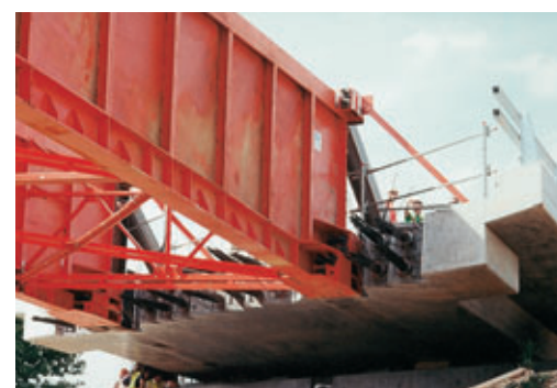
Photo 3 Avant-bec en about de tablier Cutwater on end of deck section
