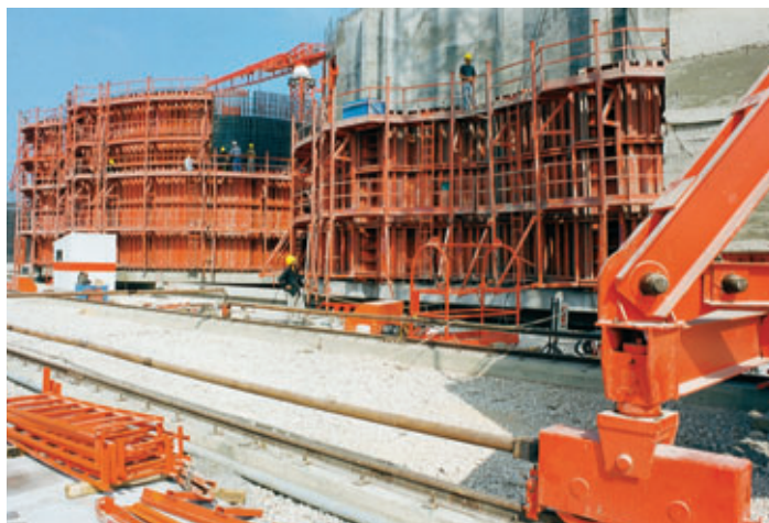
Photo 6 Caissons en stations 3 et 4 Caissons at stations 3 and 4
