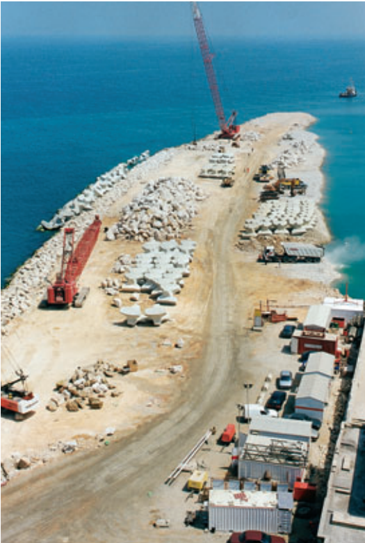
Photo 13 Western Breakwater Western Breakwater
