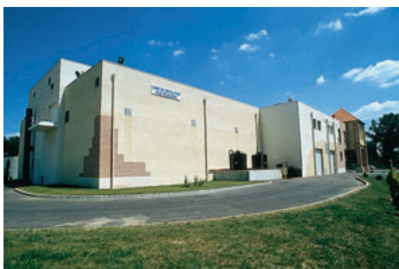
Vue générale de la station General view of the station
