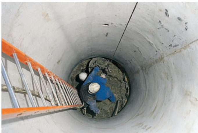
Photo 2 Havage DN 1500 Undercut pipeline of 1,500-mm ND
