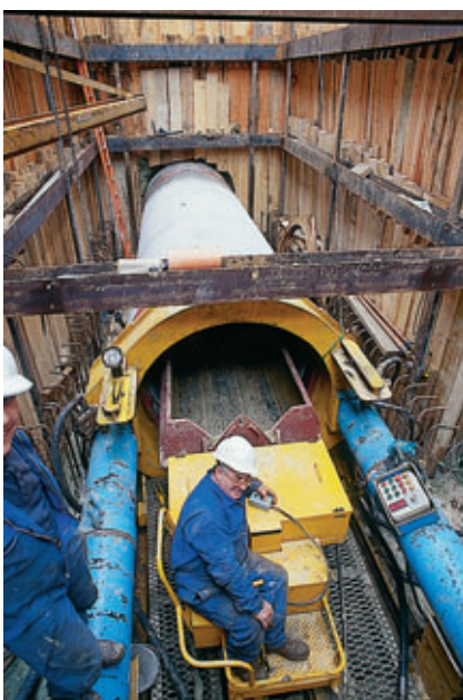
Photo 4 Installation de poussage Forepoling installation
