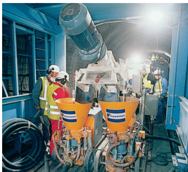
Atelier de projection sur train-travaux Spray plant on work train
