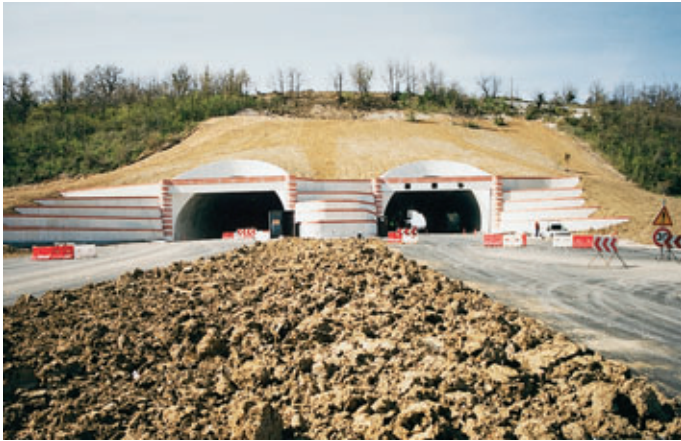
Photo 3 Têtes sud terminées South heads completed
