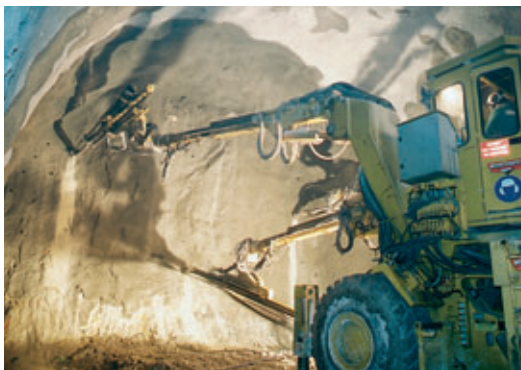
Photo 2 Le robofore en action The Robofore drill in action
