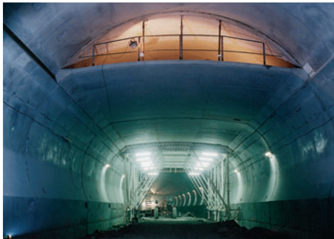
Photo 8 Dalle de ventilation Ventilation slab
