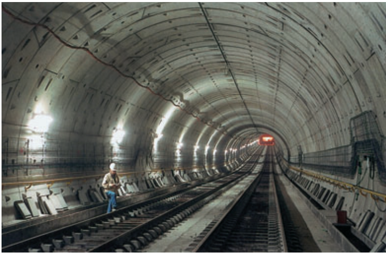
Photo 5 Aspect du tunnel terminé View of achieved tunnel
