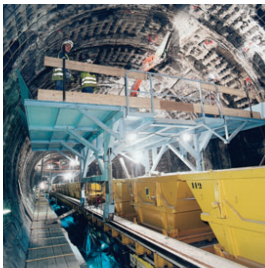
Equipements du train-travaux Equipment of work train
