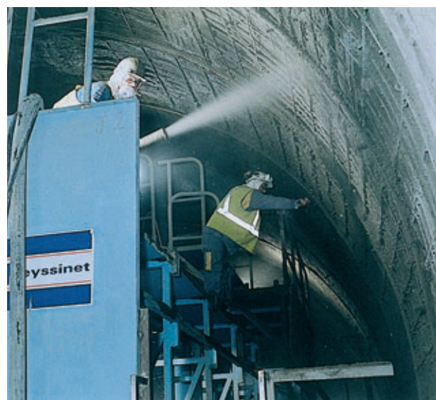
Projection du béton de restauration fibré Spraying of fiberised restoration concrete
