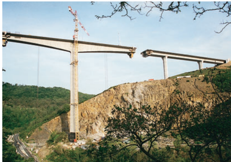
Photo 8 Fléau haubané Cable-stayed cantilever arm
