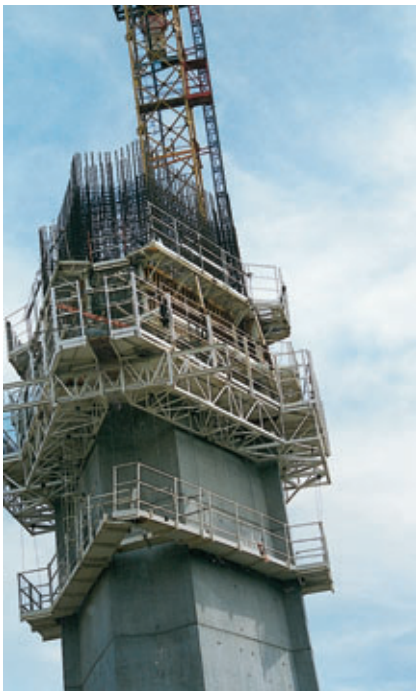
Photo 5 Le coffrage grimpant des grandes piles Travelling formwork for large piers
