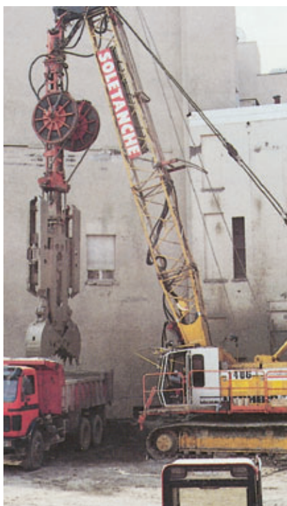
Photo 2 Outillage KS 3000 en bordure de mitoyen KS 3000 tool against adjacent structure
