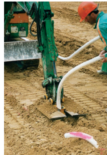
Photo 1 Pose des drains sous pelouse Placing of drains under turf
