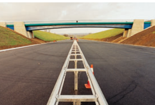
Photo 7 Couche de roulement BBTM 0/6 0/6 very thin asphalt wearing course
