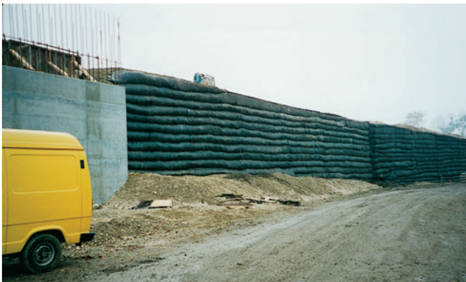
Access embankments. Geotextile and slag
