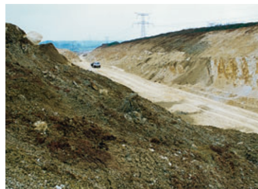
Photo 2 Terrassements section OA6 - OA7 Earthworks on section OA6 - OA7
