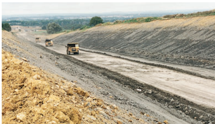
Photo 3 Terrassements section OA22 - OA23 Earthworks on section OA22 - OA23
