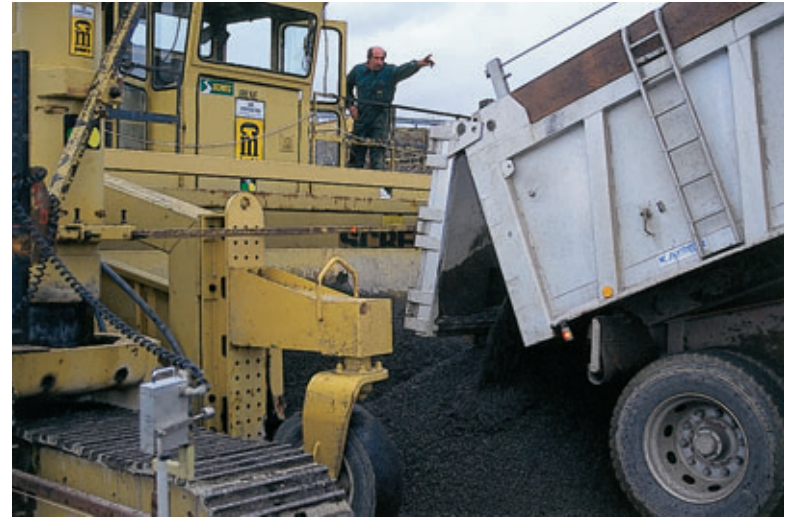
Photo 5 Application de la GRH Application of RHGM
